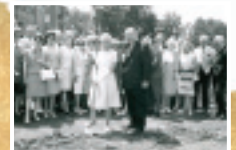
1966—Groundbreaking for Scully Natatorium
