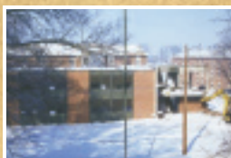
2000—Demolition of Forsyth Hall
