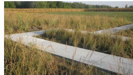
Freshly poured sidewalk into the 3-year-old restored prairie at Creekside
