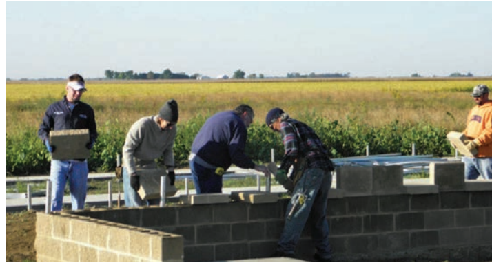
Greenhouse block wall being constructed by Friends of Creekside
